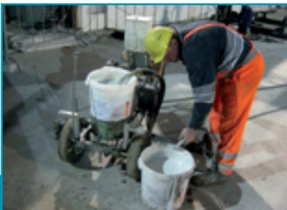
Example of a piston airless machine being used
