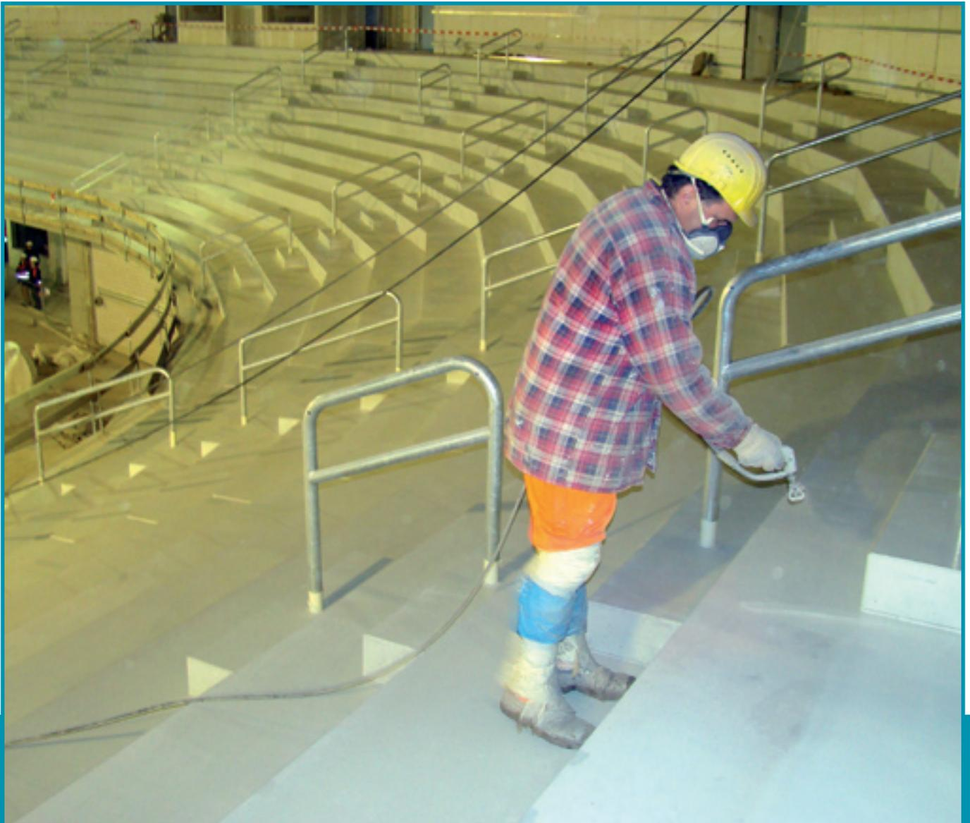
Airless spray method for ROMEX<sup>®</sup> coatings
